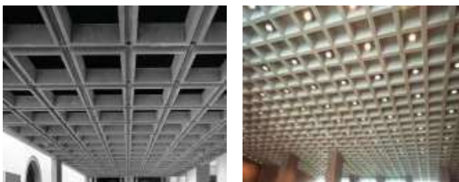
Fig-1: Grid Slab
